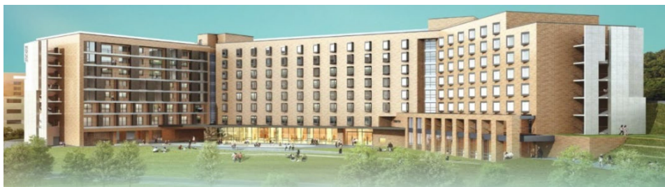
Figure 2. Chejung House (near East Gate)
